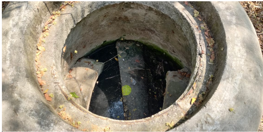
Fig 5: Manhole after cleaning
