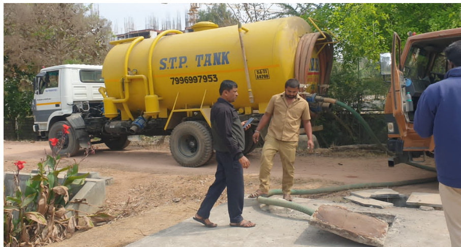
Fig 8: Sludge removal from the DTS
